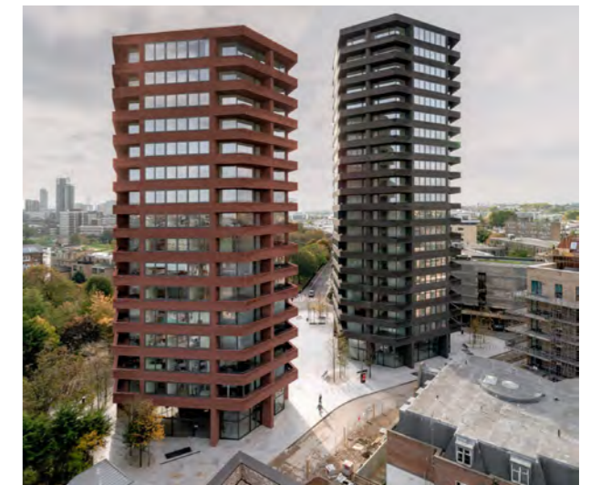
Hoxton Press, London Chipperfield Architects, 2018
